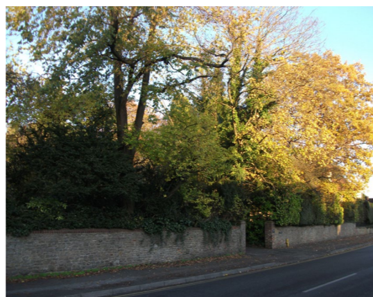
The wall on Portsmouth Road
